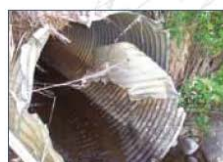
damaged culvert
