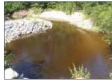
scouring and erosion
