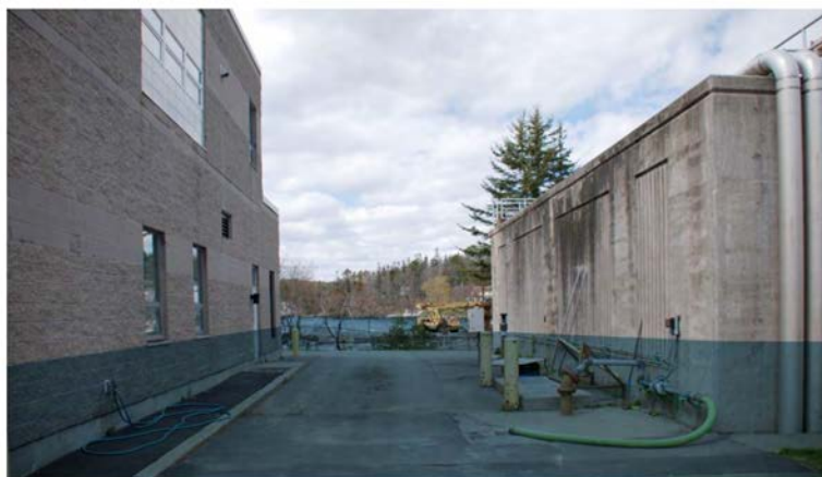
WWTP Looking North Between the Process Building and SBRs - BFE +4
