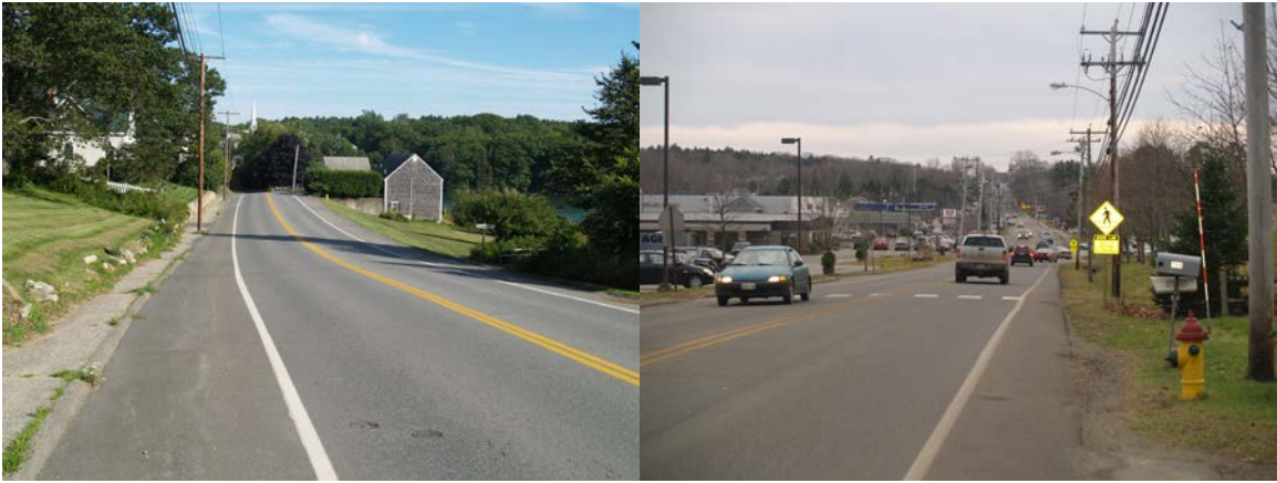
Figure 13 Variable Width Shoulders on Route 27 North of Boothbay Common
